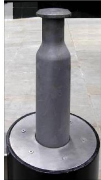
The photograph on the right shows the locking pin in the raised position but with the gate open. This is shown as an aid to understanding how the substantial mechanism, normally hidden within the gate post, is operated.
